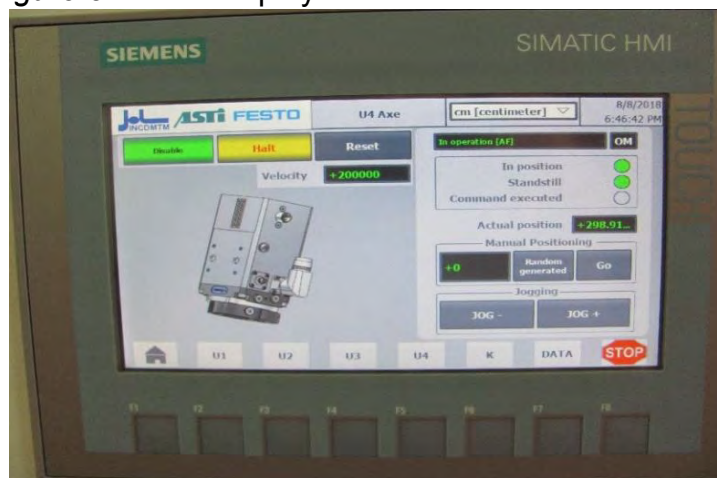
b- HMI display for command and control of the MMI4D system
